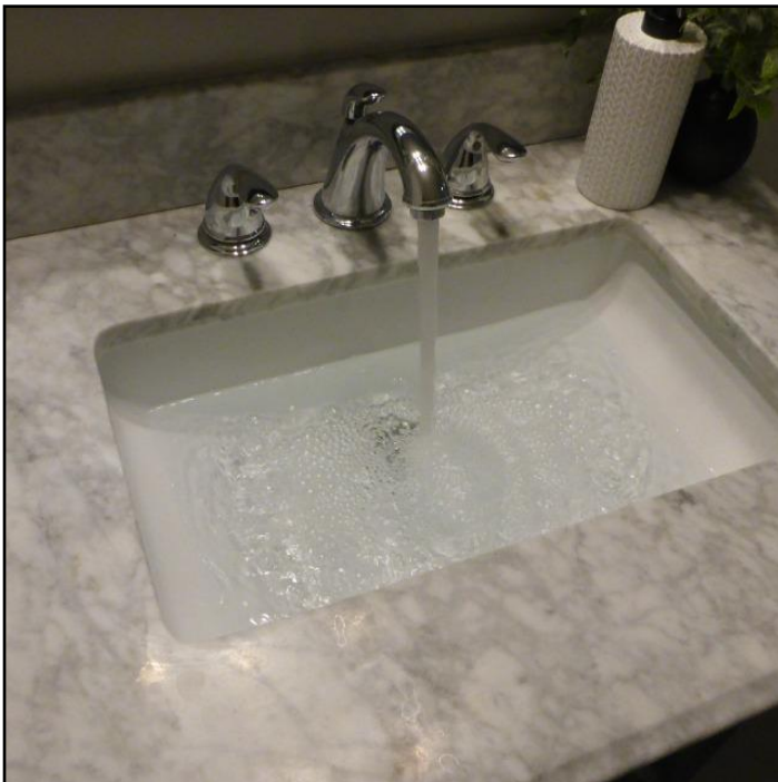
Slow drain in basement
