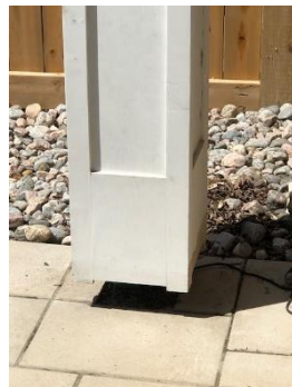
P: the ceiling/trim of the west porch overhang requires paint. The wood columns are capped with wood and some of the wood finishing that borders the posts at grade is poorly done/incomplete.
