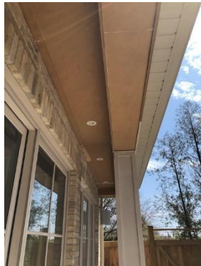
P: the ceiling/trim of the west porch overhang requires paint. The wood columns are capped with wood and some of the wood finishing that borders the posts at grade is poorly done/incomplete.
