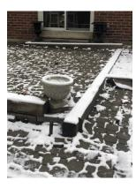
G: relay the interlocking bricks in front of the rear sliding door set and replace the wooden ties that border the rear paving stone patio as they are rotted/uneven.
