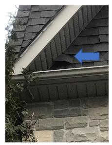
*G:* secure lifted shingle on front gable at southwest corner. As well, there is a shingle that has loosened at the northeast corner on the mansard roof- below the upper roof structure.
