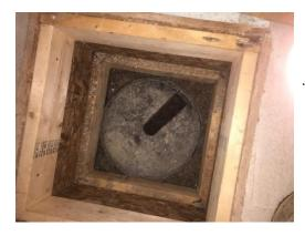
*M:* there is a sump pit in the basement floor near the electrical panel. These are typically installed to deal with foundation waterproofing systems. As the basement is located at or above grade, the need for foundation waterproofing would not have been required. The pit in the floor has some groundwater present, as would be expected. There is no sump pump present. There is no evidence that water has breached the pit and so long as this continues, a pump would not be required.
