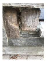
G: there is localized mortar loss between stones on the front deck that should be repaired.
