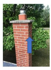
*G:* at least two bricks have lost their protective outer facing, exposing the soft inner core of the brick to the elements (known as spalling). A couple of others are cracked. The damaged bricks should be replaced. (Approximate Cost: \$500 to \$800)
