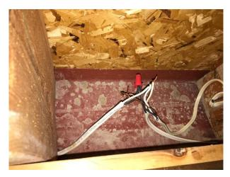
*P: unprotected wiring connections are visible in the two locations in the basement ceiling. One is located near the steel I-beam in the NW basement utility room. The other is located on the doorframe opposite the furnace. The wires should be reinstalled in a junction box to prevent them from becoming loose.*
